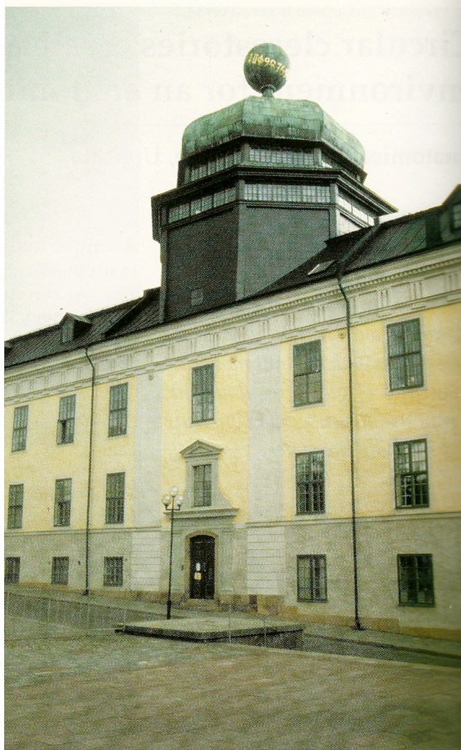
△ Exterior view showing the two rows of clerestories.
